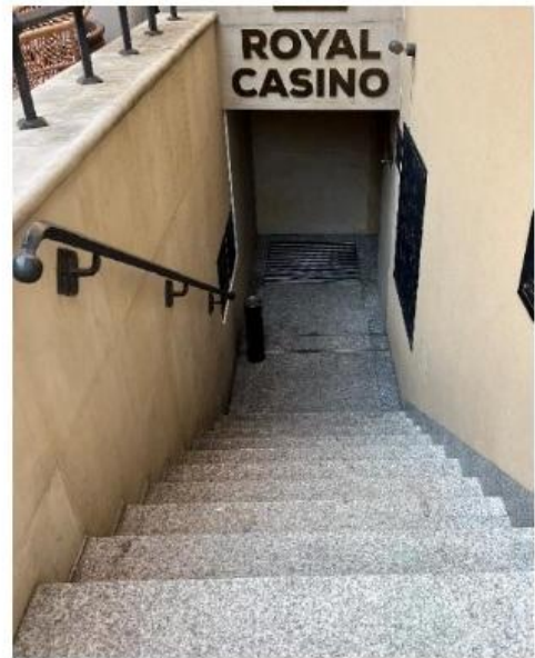
Fig. 8. Smooth stair surface with handrail; Source: Author
